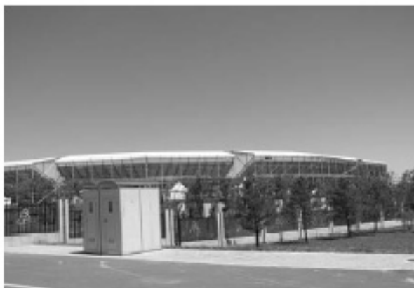
(b) Picture after installation
