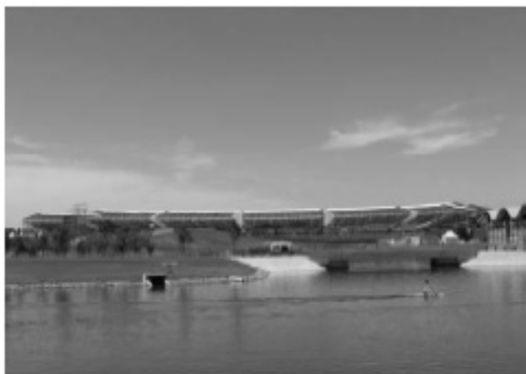
(a) Picture before installation
